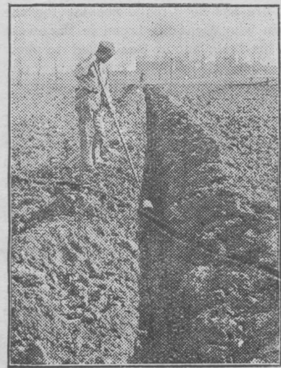
POOR WAY TO LAY TILE.
