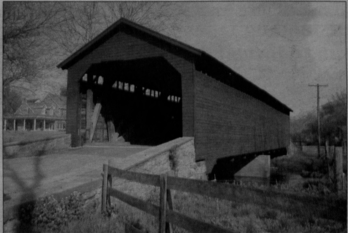
Utica Mills Covered Bridge
