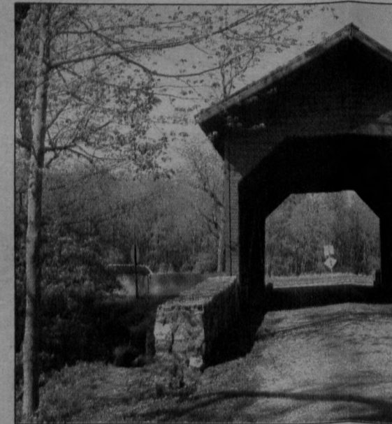
Roddy Road Covered Bridge
