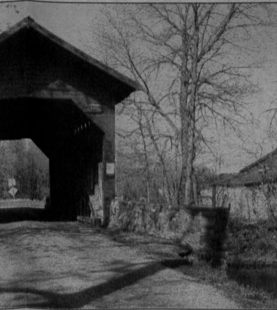
oad Covered Bridge
