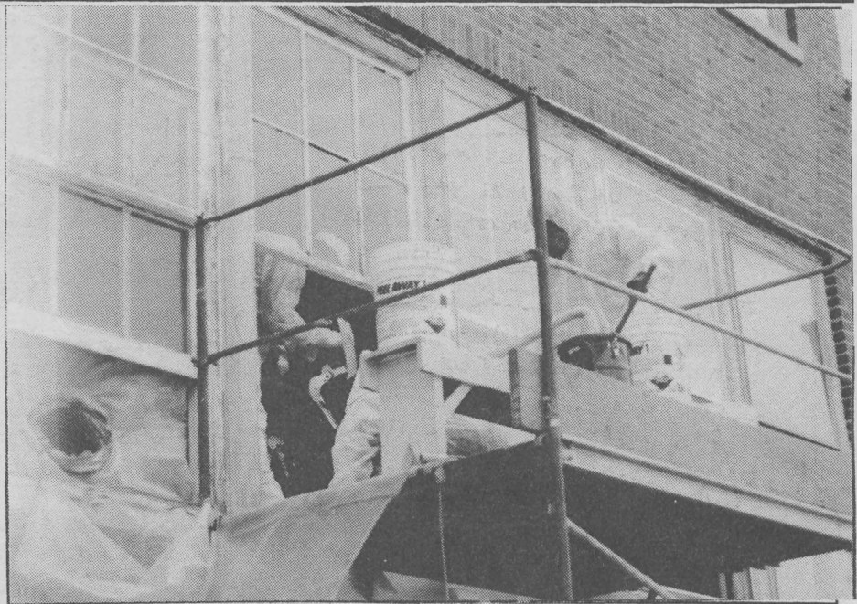
Men from Mars assist county in "getting the lead out." The Hazmat Abatement crew from Envirabat clean up lead paint from Community Center windows. A Dispatch Photo
