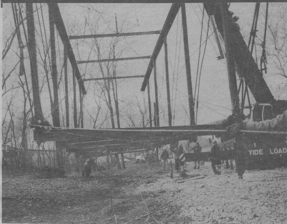
The Four Points Bridge comes ashore.
