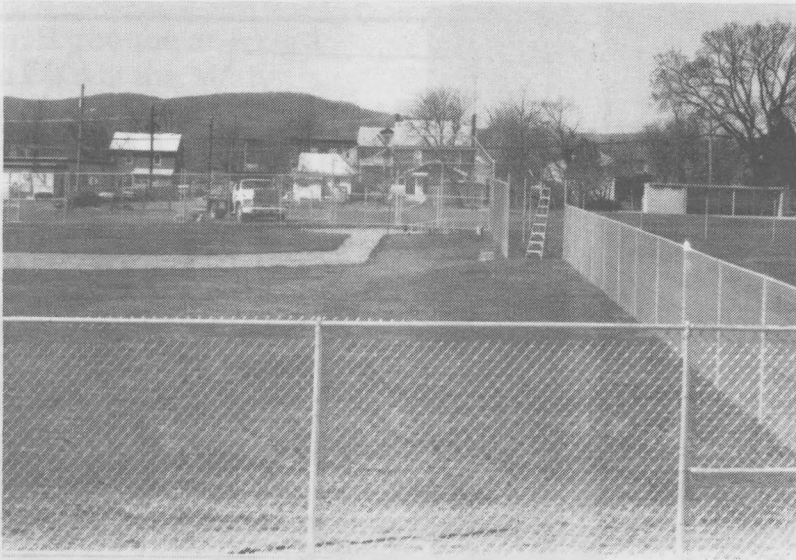
Memorial Park— New Little League fields under construction A Dispatch Photo
