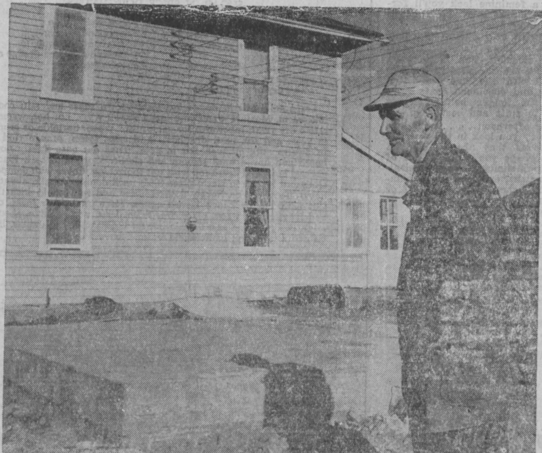
SURVIVAL INSURANCE looks like an ordinary concrete slab at the home of Don S. Trow near Albany, Wis. But beneath the slab is a $1,500 reinforced concrete shelter which the 68-year-old farmer ordered built for himself and his wife. Trow got the shelter plans by writing to Box Home Shelter, Office of Civil and Defense Mobilization, Battle Creek, Mich. (Wisconsin State Journal Photo)
