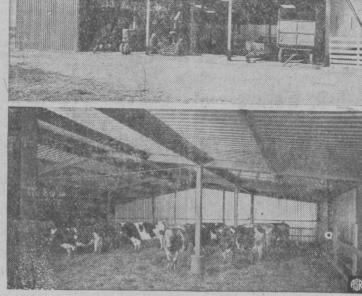
A new concept in steel buildings for livestock shelter and machinery storage has been achieved with a pre-engineered all-steel pole lavilding that can be erected by the owner himself.
