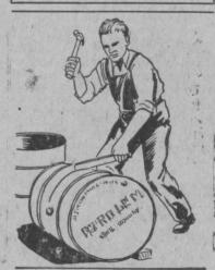
The problem of cutting discarded oil drums for various farm uses may be solved by using an old corn knife and hammer. Hold knife so that about 2" of blade is inside drum, apply hammer blows as close to cutting point as pos-
