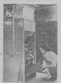
Basement-located forced warm air furnace doesn't take up much room. Photo shows filters being changed, a job easily accomplished by owner.
