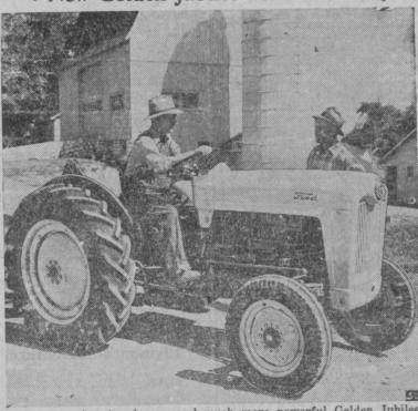
A new, heavier, longer and much more powerful Golden Jubilee Model tractor has been put into production by the Ford Motor Company, manufacturer of more than two million farm tractors since 1917. The new machine is described as the most modern farm tractor ever built. It has new advanced hydraulic controls and is powered by an entirely new overhead valve Ford "Red Tiger" engine. In 1953 the company celebrates the 50th anniversary of its founding by Henry Ford Sr., in 1903.
