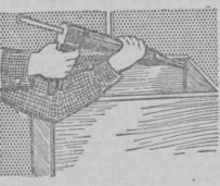
to putty (not wood putty) but never becomes hard or brittle. This compound is much used for repairing outside leaks around window frames. It is forced into the crack with a caulking gun. Inquire about this at your hardware store.
