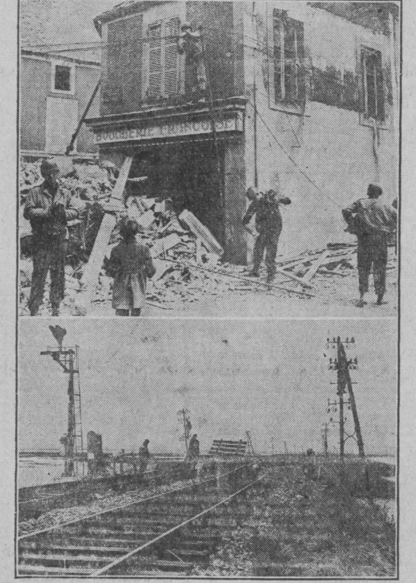
(Upper) Working under extreme hardship, Signal Corps men string wire to establish communications in Trevieres, France, after the town was occupied by American troops. Rubble in the streets resulted from aerial bombing and gunfire loosed on the town prior to its occupation by the Americans. (Lower) Retreating Germans shattered telephone lines in blowing up the above railroad bridge somewhere in France, but Signal Corps men were right on the job afterwards to make speedy restorations. The Germans also flooded the surrounding area, as shown above.
