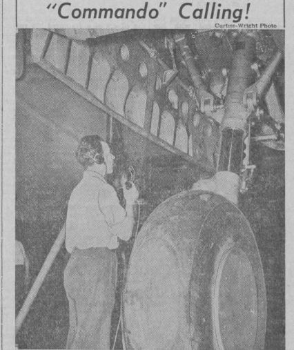
So big is the Curtiss Commando, giant new U.S. Army air cargo carrier, that workers employed on pre-flight checks are equipped with Western Electric telephone headsets for inter-communication. Thus, despite the din of shop noises, this testman can report responses of the huge hydraulic landing gear to controls operated by a fellow worker in the cockpit.
