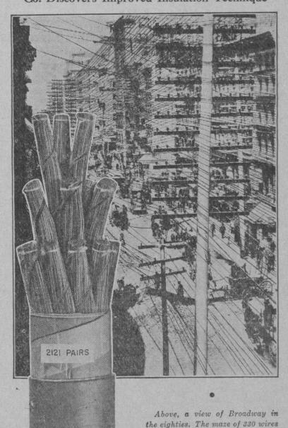
development of lead covered telephone cable, engineers of the Bell System have made another historic advance with the manufacture of cable containing 4,242 separately insulated copper wires. Heretofore, the maximum contained in one cable was 3,636 wires. Despite the increase in the number of wires, the new cable is no larger around than its predecessor, its diameter being exactly the same-2%
