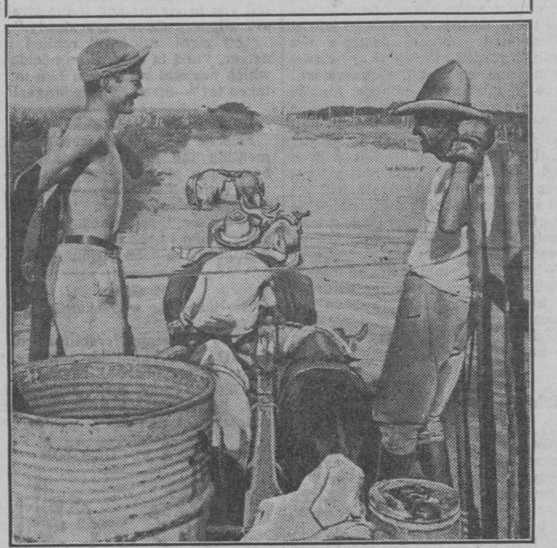
Transporting the equipment for drilling the dynamite shot holes. Firing of the dynamite creates sound waves which aid in exploring the earth's subsurface.
