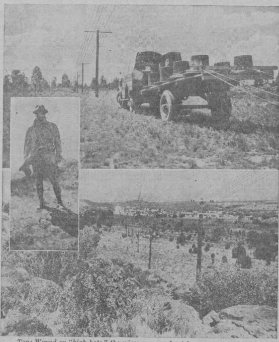
Top: Wound on "high hats," the wires are payed out from a motorized hat rack as the linemen advance across the country. Bottom: A section of the fourth transcontinental telephone line near Ashfork, Ariz. Insert: Photo showing member of survey crew equipped with goggles and mask. These were regular items of equipment during the dust storms last spring.
