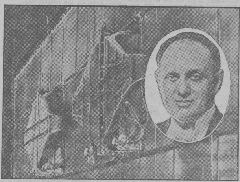
Rear curtain view of new shallow loud speaker horns developed for sound picture theatres. Inset, Roxy, in whose theatre these horns are used.
