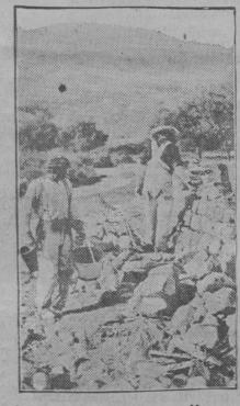
Construction of Cobblestone Masonry
