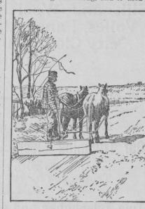
DRAGGING A ROAD. the right time one man and three horses will do more and better work with it than three men and six horses can do with an expensive road grader, working, as is the custom, at the wrong
